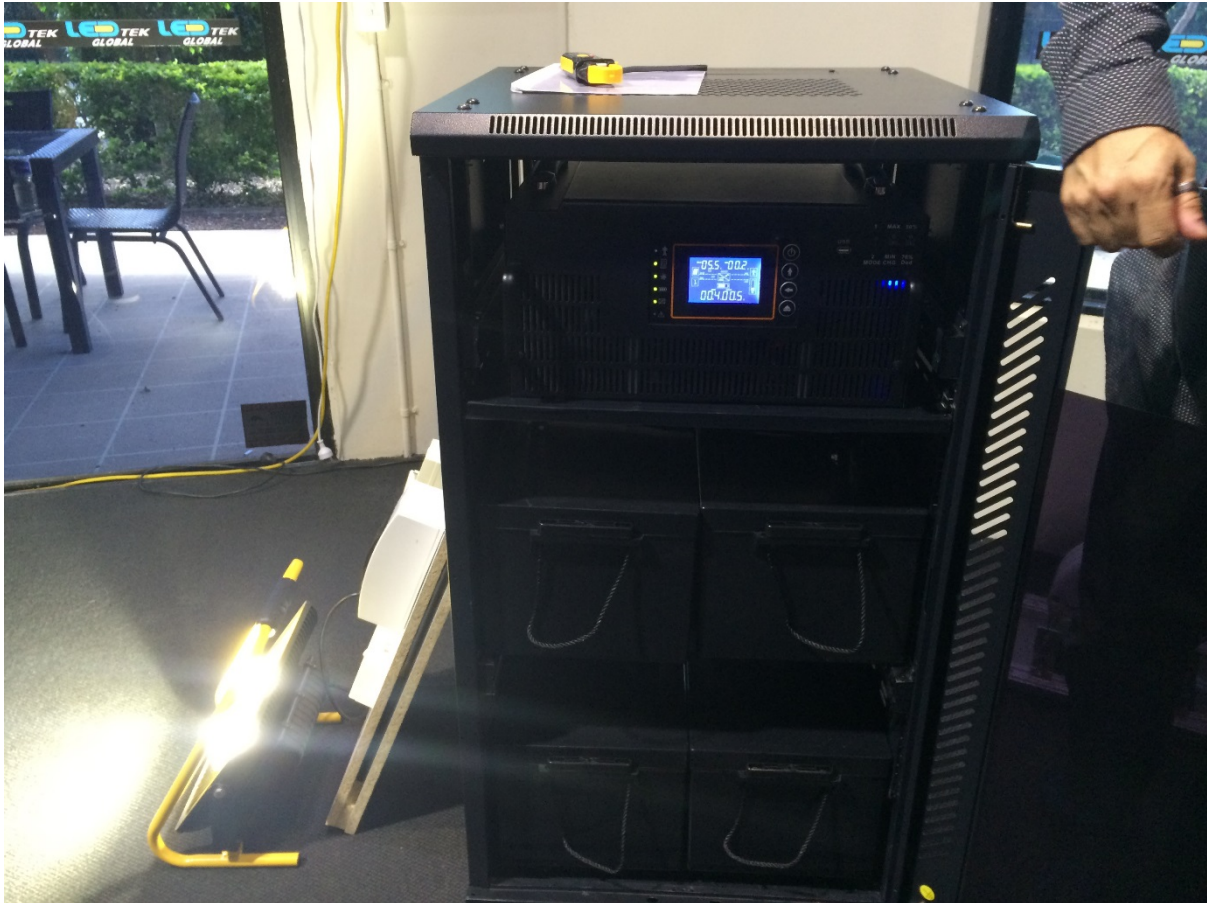
With PV connected and battery is supplying the load
